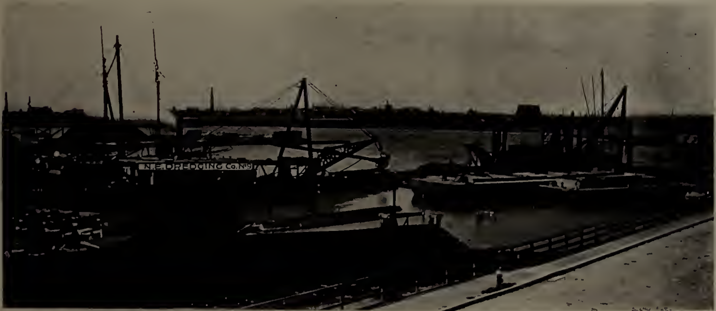
NEW ENGLAND DREDGING COMPANY'S SCOOP DREDGE NO. 9 IN OPERATION. Office, 12 Post Office Square, Boston.
